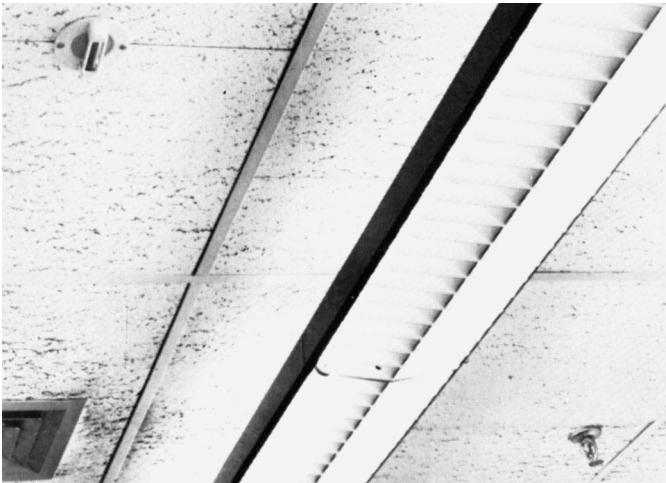
Figure 5. Typical ceiling installation of a horizontal DETECT-A-FIRE model. Here it is used in combination with a sprinkler system to detect overheat and actuate an alarm.
